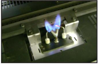
Figure 3.1 IPI Pilot Flame Pattern
